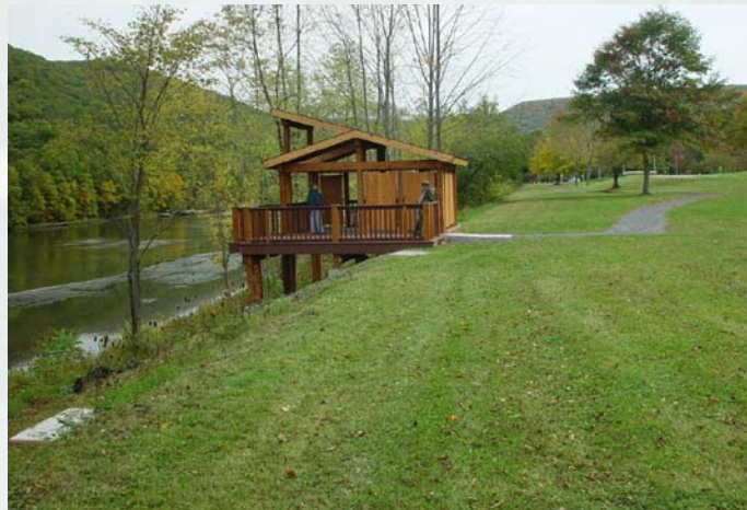
Completed Riverside Watchable Wildlife Viewing Platform and Trail Kinzua Dam and Allegheny Reservoir
